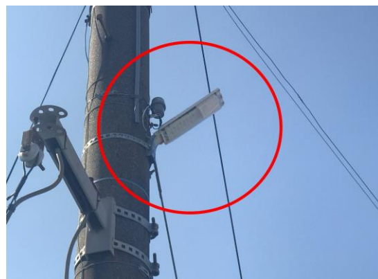
After No.635 LED 街路灯の新規設置 (登町)
